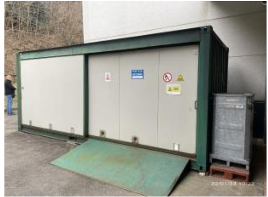
Chemical products storage (external)..JPG
